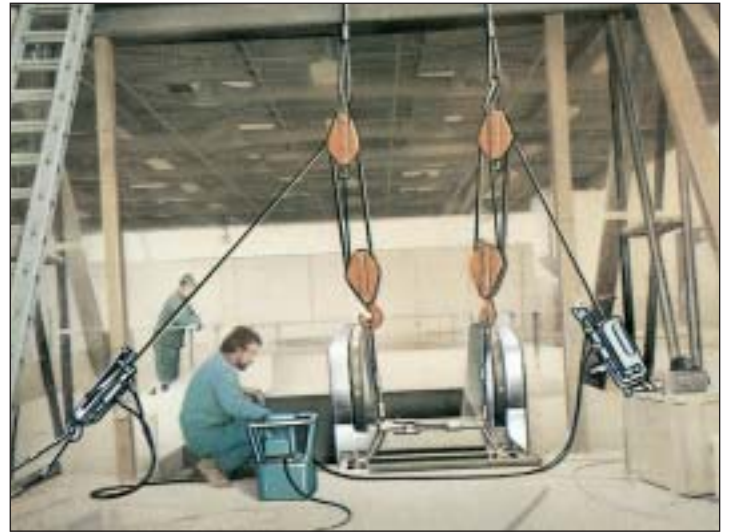
2. Fig. 3 – Installation of a mechanical escalator (TU-16H).
