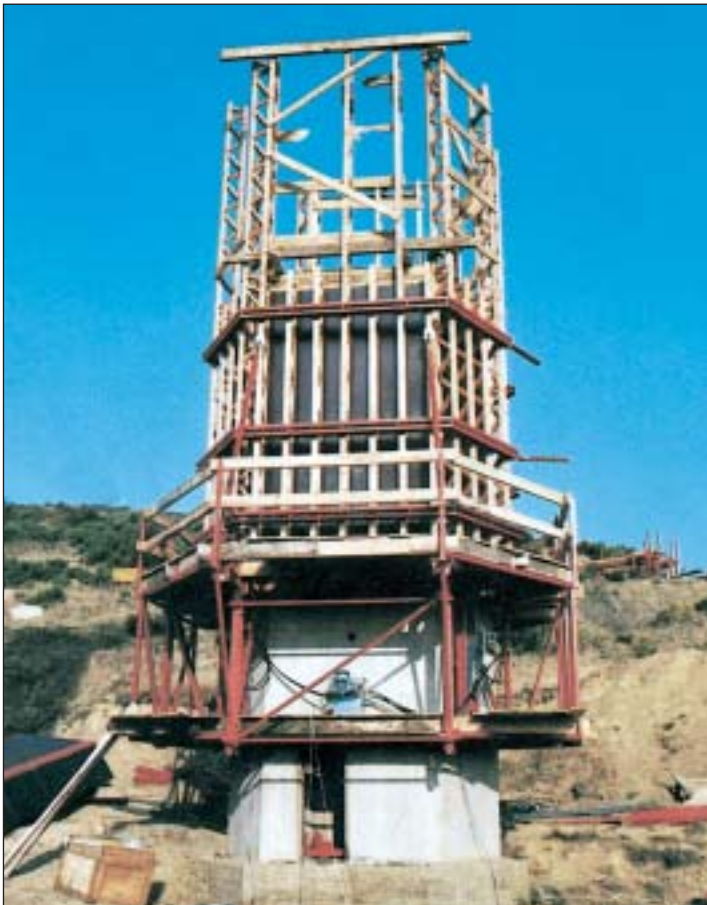
Fig. 2 – Operation of self climbing shuttering, PERI system (TU-32H).
