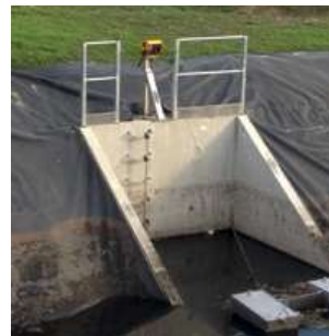
▷ Opening of a sluice gate.
